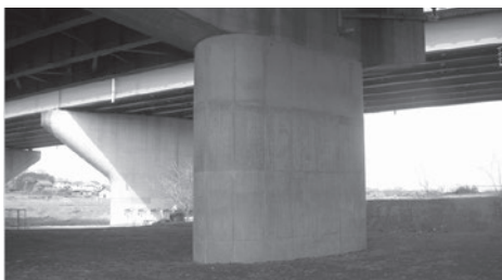
耐震補強施工後
